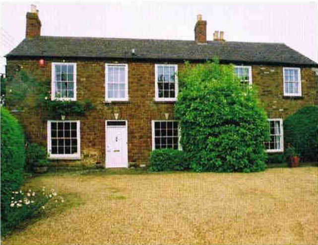
Figure 10.14c: Front of Old Vicarage at 65 Church Street
