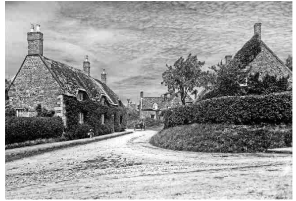
Fig. 1.5: Revells Corner, Church Street
