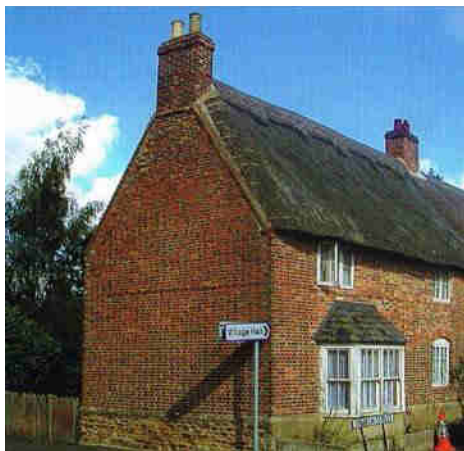
Figure 10.6: Flemish Bond at 22 Church Street
