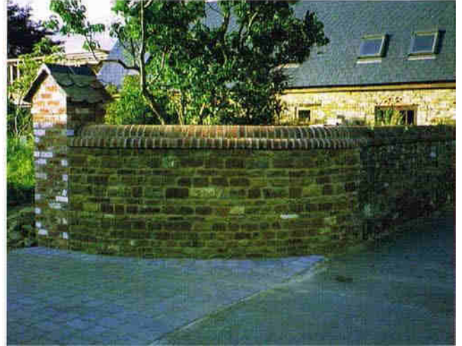
Figure 10.14b: Yew Tree House entrance on Burley Rd
